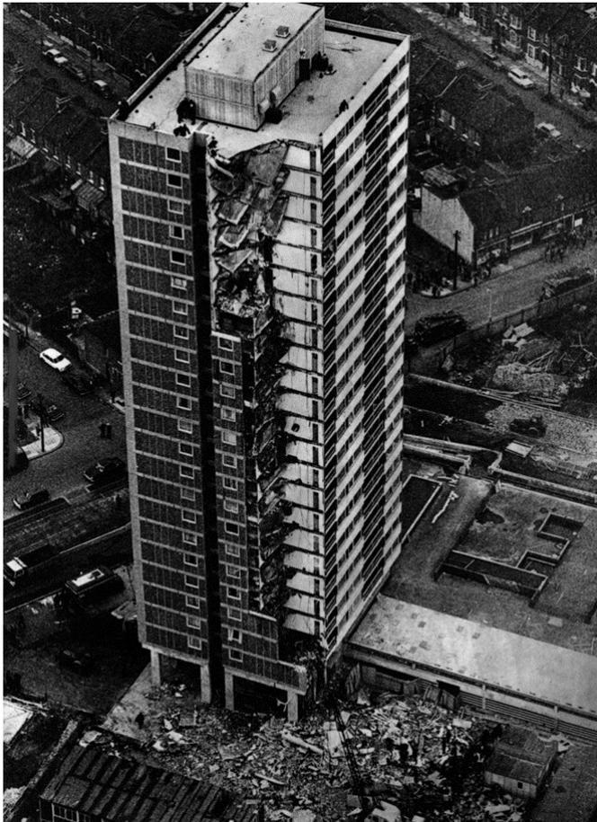
**Figura 31.** Collasso Roman Point (<http://www.failedarchitecture.com/the-downfall-of-british-modernist-architecture/>).
