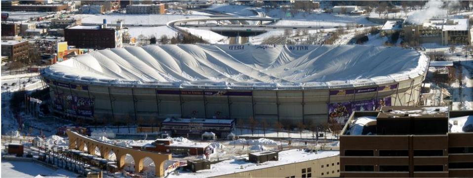
**Figura 12.** Minneapolis Metrodome Collapse.
